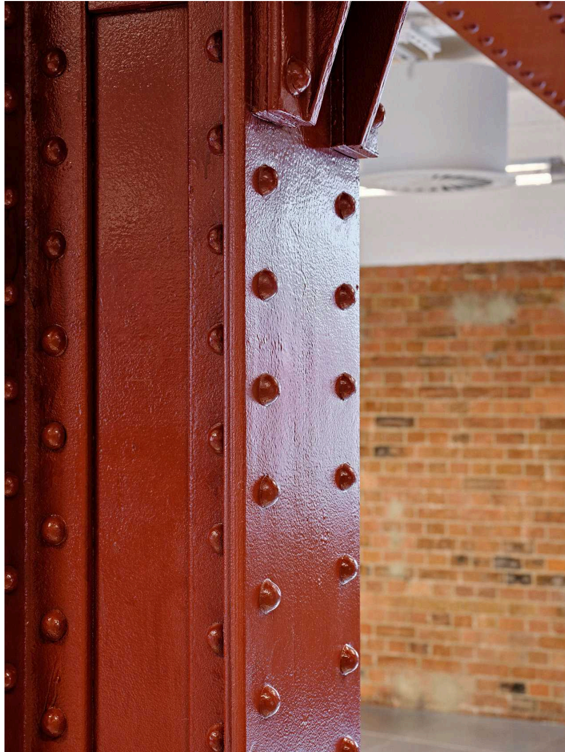
Retained steel columns
