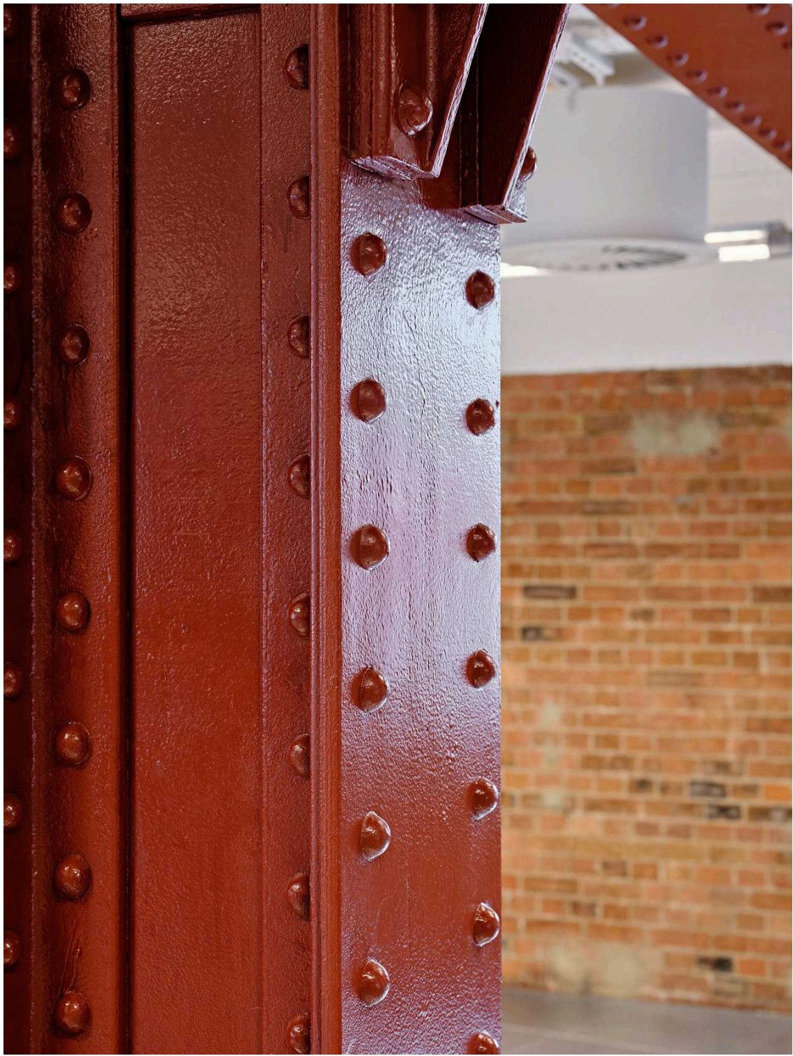
Retained steel columns
